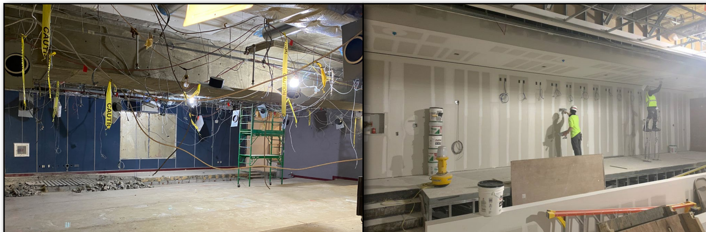
Removing outdated and analog technology and wiring was necessary to modernize the Training Center.
