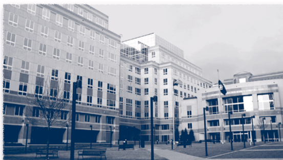
Expansion of Virginia Square Facility
